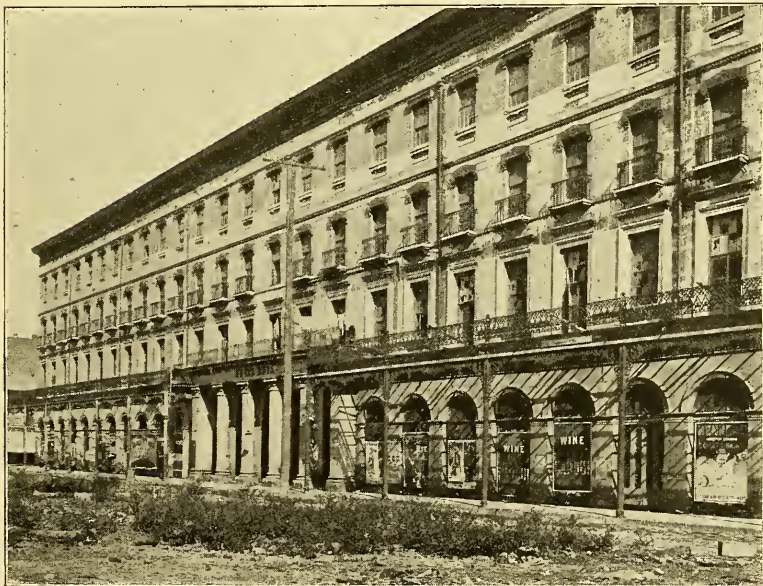
Old Hotel Royal, recently demolished —See Page 36.
